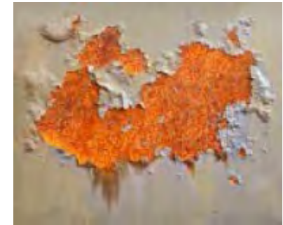
Corrosion protection coatings
