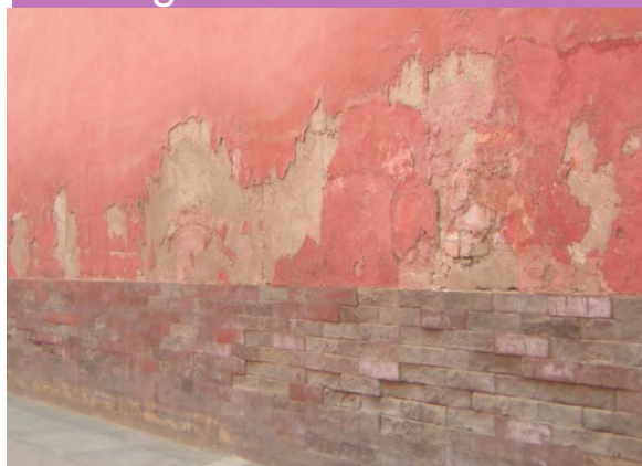
Ingress of water leads to damage of facades
