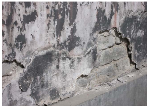
Ingress of water leads to damage of facades
