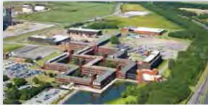
National Industrial Biotechnology Facility
